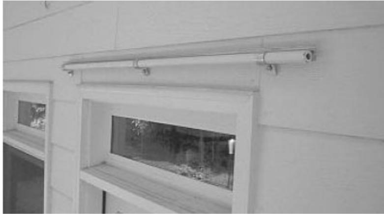
Ensure the back bar is level and fasten the clamps tightly to the wall.
