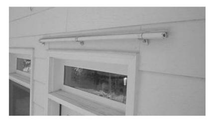
Ensure the back bar is level and fasten the clamps tightly to the wall.
